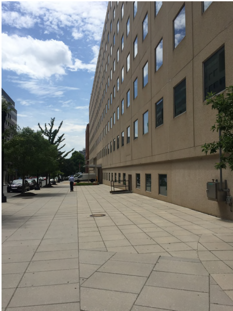
1. F Street View, SE View
