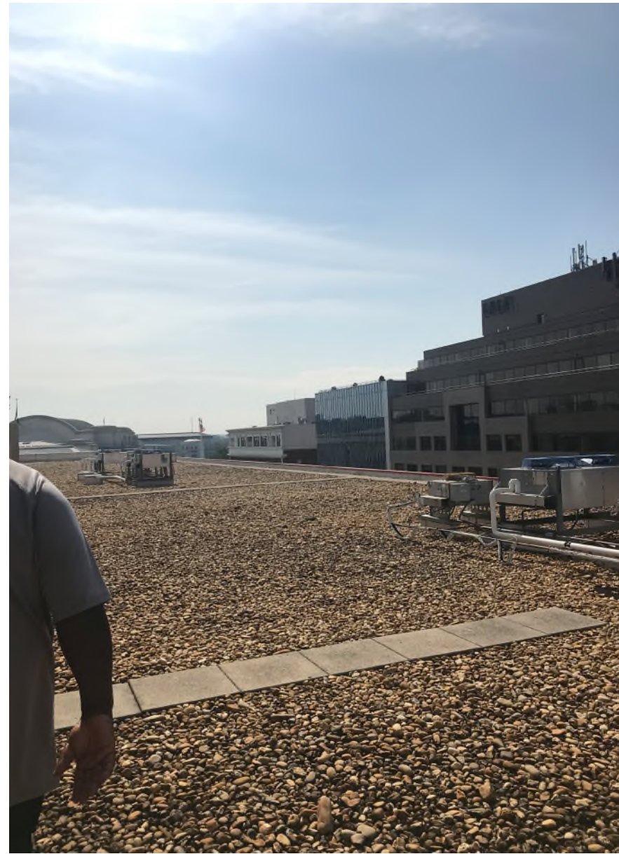
2. SE View from Roof
